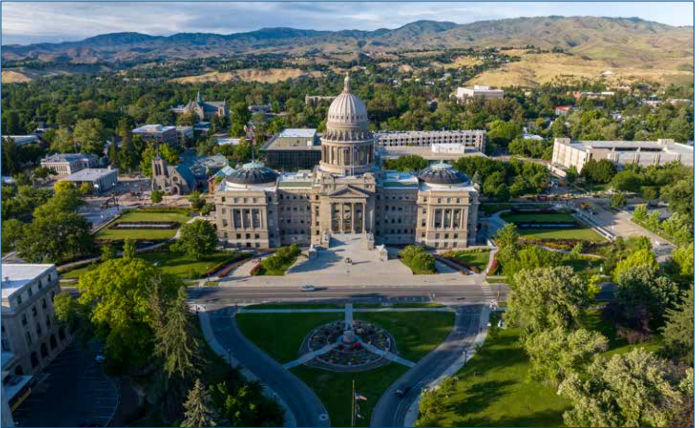
The Idaho State Capitol building in Boise
