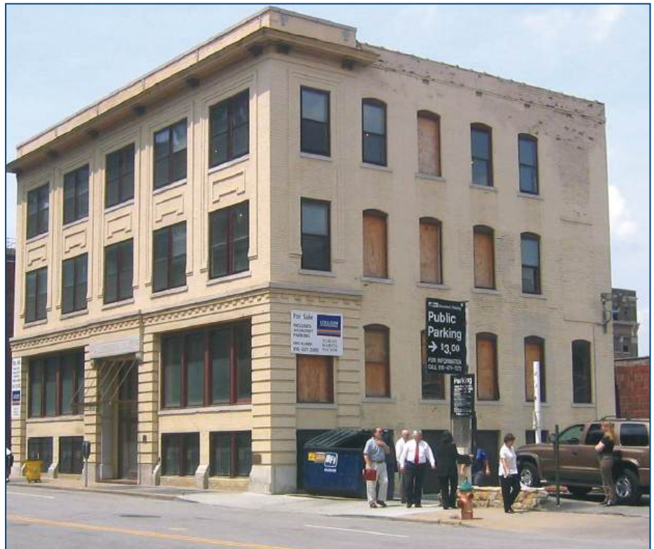
IAAO's Adler Building in downtown Kansas City ...
